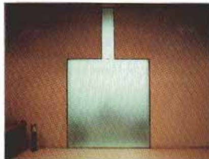
FIGURE 3-28 Only light is exchanged between the corridor and office space in the addition to the Banco Popolare (Carlo Scarpa, 1973–81) in Verona, Italy. The obscure glass maintains visual and acoustical privacy for office workers. Photograph by Lucy Carter Sloman, ©1996.
