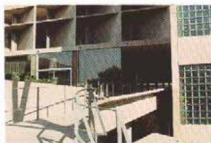
FIGURE 3-15A Le Corbusier's vocabulary of window forms on the west façade of the Carpenter Center for the Visual Arts: pans-de-verre , aérateurs , and brise-soleil .
