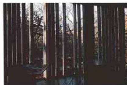
FIGURE 3-15B View from inside the north-facing studio showing ondulatoires and aérateurs . Photograph by Ronald Kellert.
