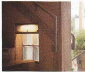
FIGURE 3-27B View of window in stairwell.
